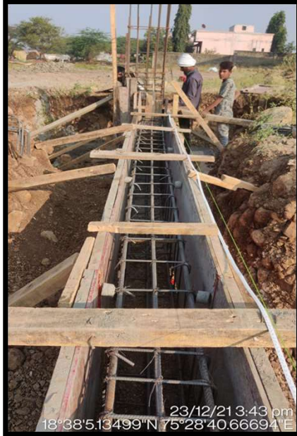
Ground beam Reinforcement & Shuttering
