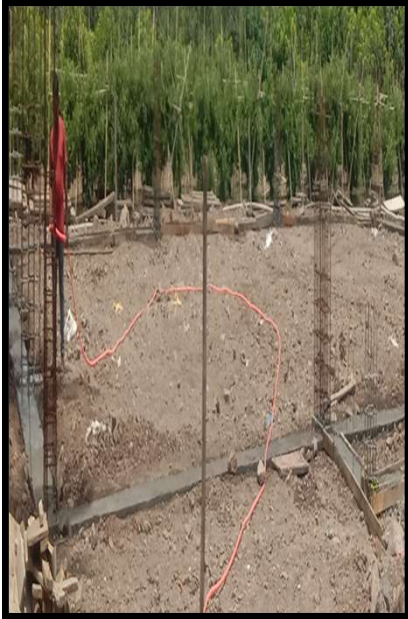
Ground beam PCC
