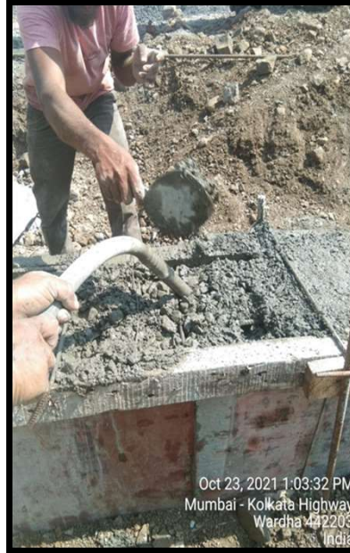
Plinth/Ground Beam Concreting
